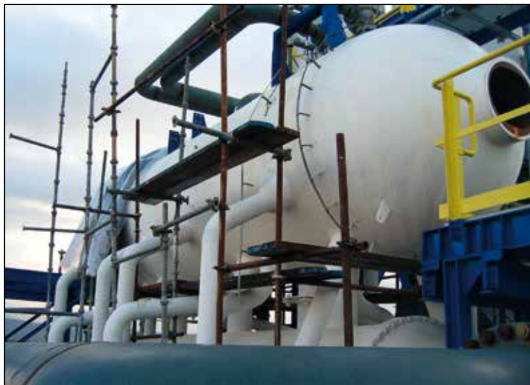
Secondary Transfer Line Exchanger / Steam drum Unit
