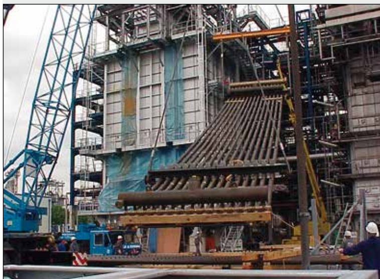
Installation of BLQ
