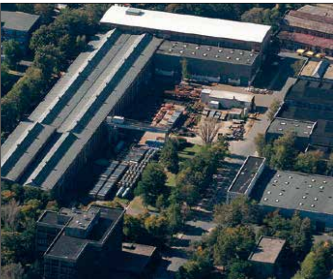
BORSIG Process Heat Exchanger GmbH workshop in Berlin
