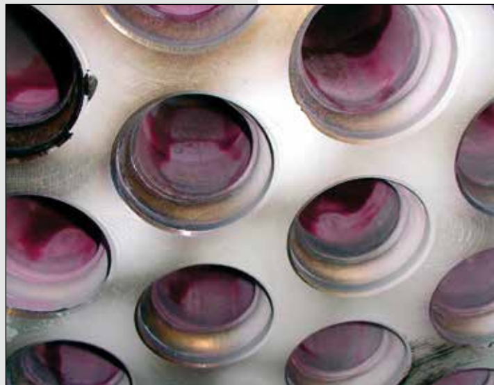
Penetration testing of TLE
